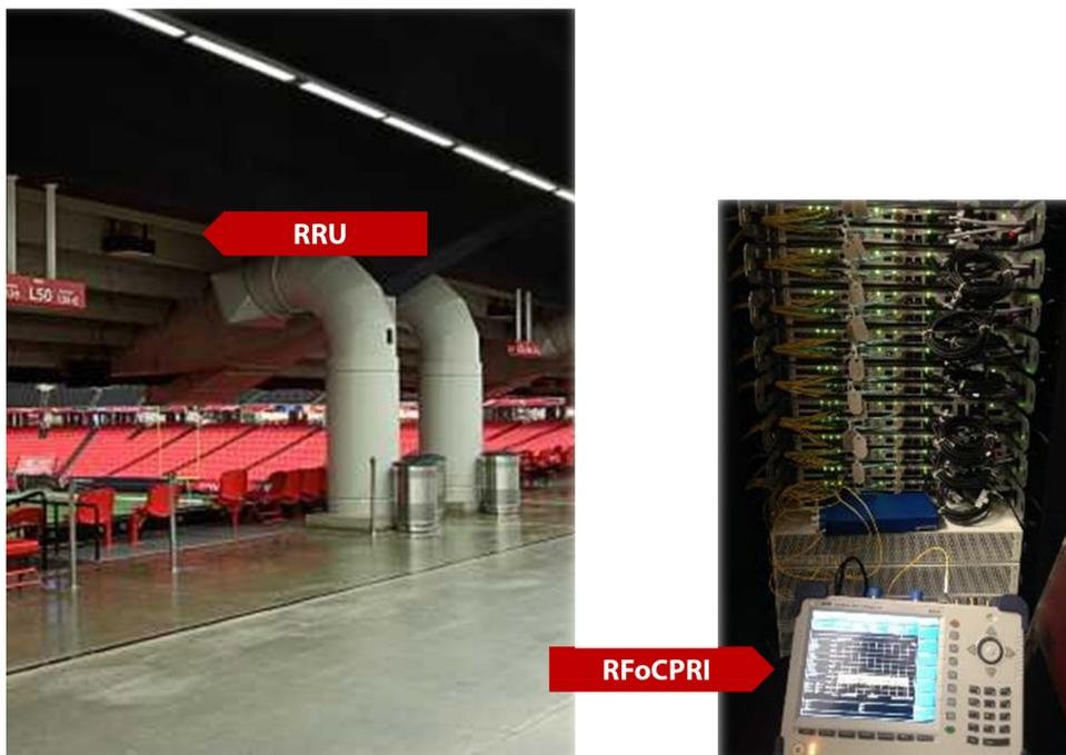
Figure 27. Distributed antenna system (DAS) and CellAdvisor with RFoCPRI
