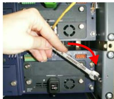
**Fig. 20** Spacer onto the OTU-8000
