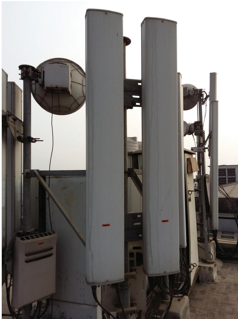
Figure 2: External PIM due to hardware issues caused by cable and antenna system
