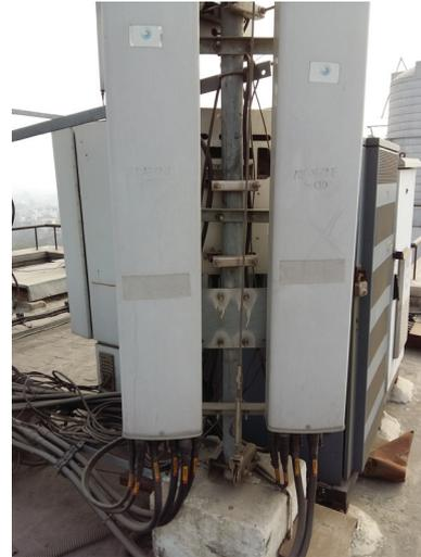
Figure 3: PIM generating antenna
